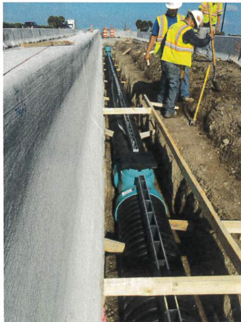
Figure 15A Duraslot Slotted Drain Pipe Installation
