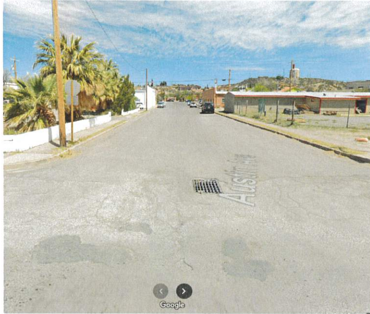
Figure 15: Existing Grate at Austin Street and Daniels Street Intersection looking North towards North Broadway Street
