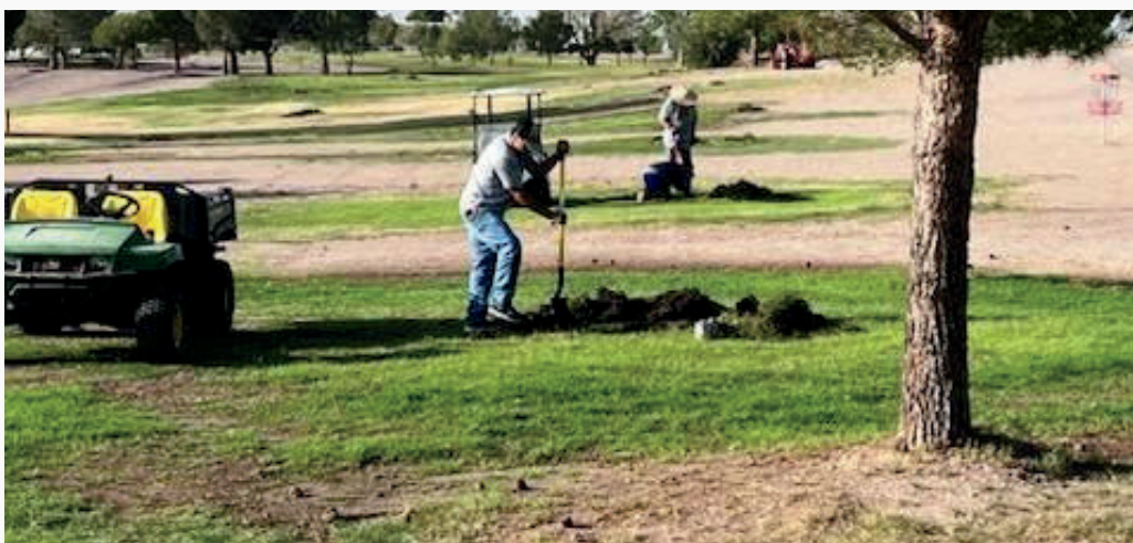
Digging up sprinklers
