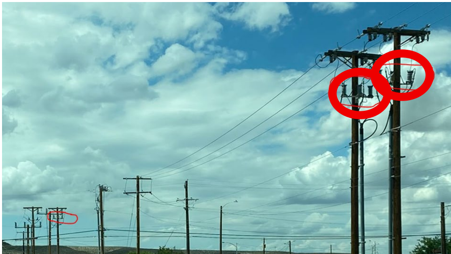
Upgrade surge arresters to polymer station-class
