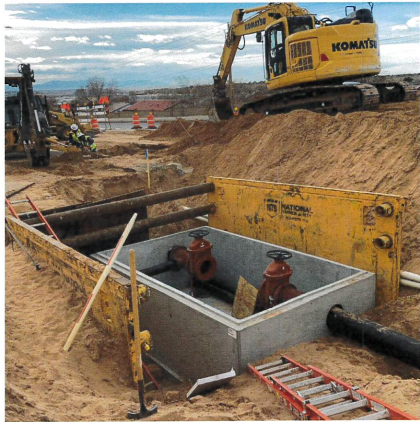
City of Rio Rancho Road Project
