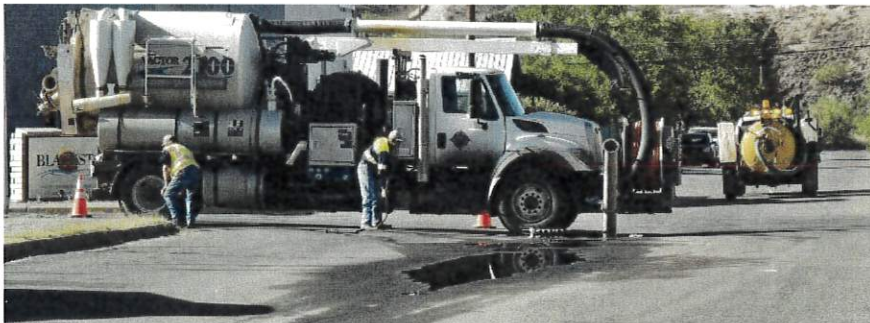
Street Crew repairs a leak
