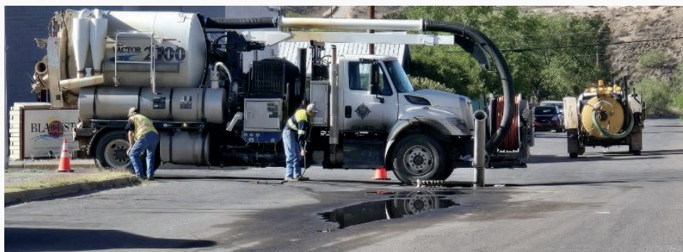
Street Crew repairs a leak
