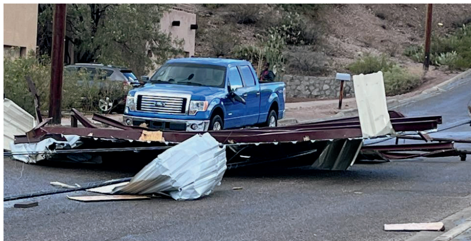
Roof debris on Pershing Street
