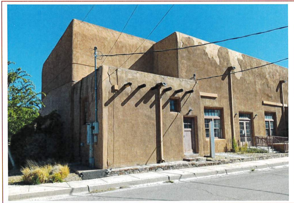
View of the building from the southwest property corner taken on April 10, 2024.
