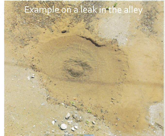
Example of a leak on Veater
