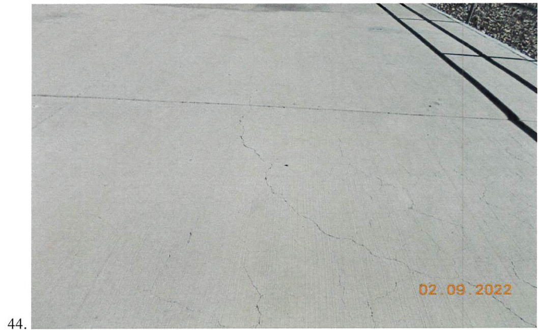
Images 41 through 44: Examples of damaged (spalled) concrete on the parapet walls of the main dam and shrinkage cracking on the crest of the main dam. Repair of the spalled concrete is required along with monitoring and documentation of the shrinkage cracks over time.
