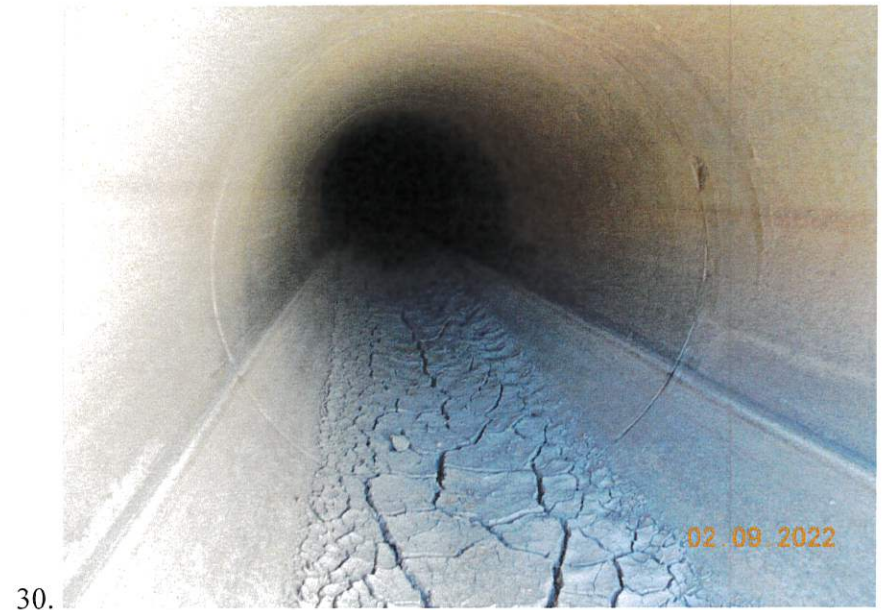
Images 29 and 30: Upstream interior views of the low-level outlet conduit as seen from the discharge end of the conduit. The upstream end of the conduit is located at the upstream face of the dam and within the outlet works structure shown in Images 26 through 28.
