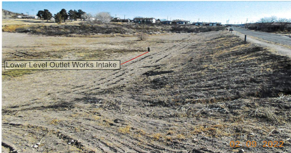
Image 7: Easterly view of the upstream slope as seen from the vicinity of the right abutment with the location of the lower level outlet works intake as indicated.
