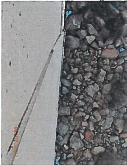
Images 47 through 49: Examples of offset joints and cracks on the upstream face, crest of the main dam and upstream face of the emergency spillway ogee section that should be monitored over time.
