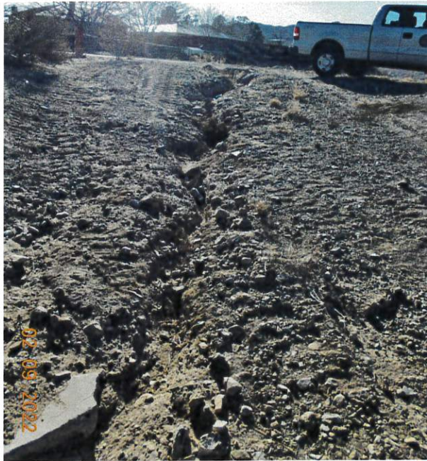
Images 21 through 23: Erosion gullies in need of repair on the upstream slope (Images 21 and 22) and more of the same on the downstream slope (Image 23).
