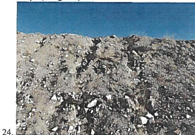
Images 24 through 26: Additional views of erosion on the downstream slope. A gravel/cobble mulch placed on the embankment slopes and abutment contacts at the upstream and downstream groins of the dam would serve well towards diminishing erosion.
