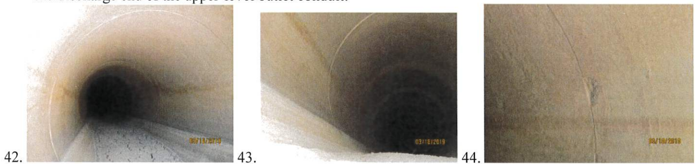
Images 42 through 44: Views of the downstream (discharge) end of the outlet works low-level conduit.
