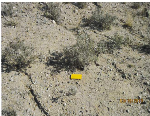
Images 11 and 12: Typical views of rodent burrows on the downstream slope.
