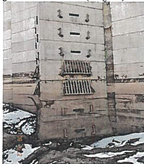
Images 26 through 28: Slightly distorted views of the low-level outlet works intake structure located at the base of the upstream face of the dam.
