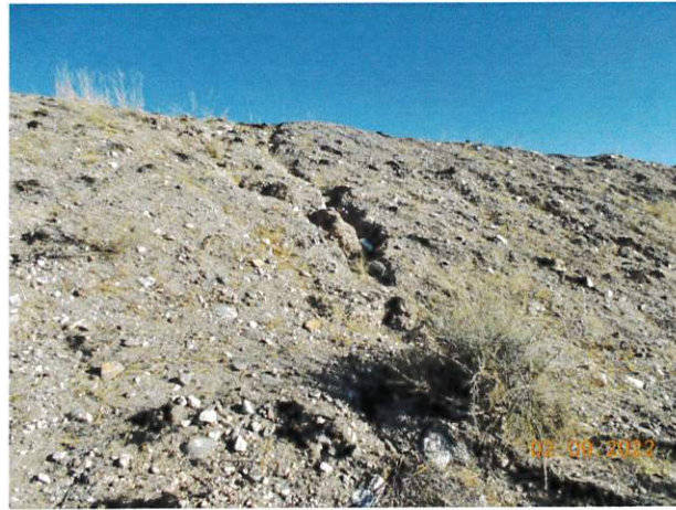
Images 24 through 26: Additional views of erosion on the downstream slope. A gravel/cobble mulch placed on the embankment slopes and abutment contacts at the upstream and downstream groins of the dam would serve well towards diminishing erosion.
