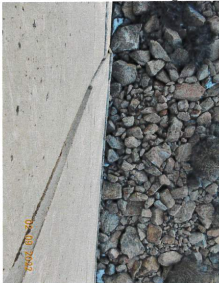
47. 48. 49. Images 47 through 49: Examples of offset joints and cracks on the upstream face, crest of the main dam and upstream face of the emergency spillway ogee section that should be monitored over time.
