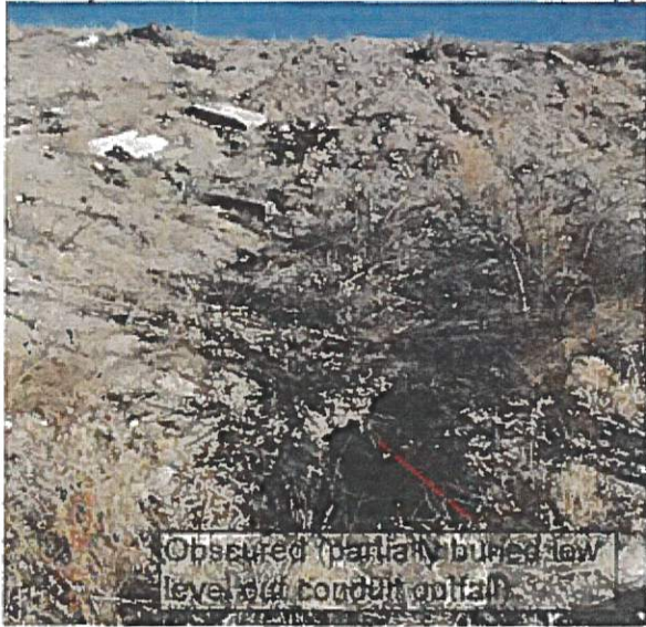
Images 13 and 14: Upstream views of the lower level outlet outfall in 2022 and 2015, respectively. The outfall is currently obscured and needs to be maintained in an exposed condition.
