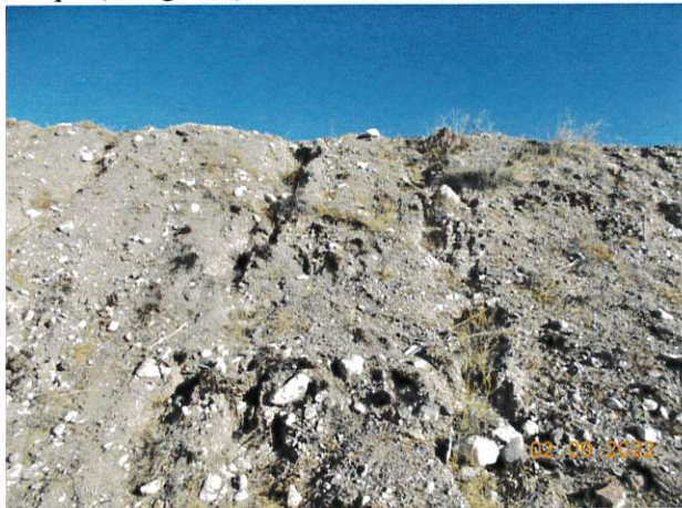
Images 24 through 26: Additional views of erosion on the downstream slope. A gravel/cobble mulch placed on the embankment slopes and abutment contacts at the upstream and downstream groins of the dam would serve well towards diminishing erosion.
