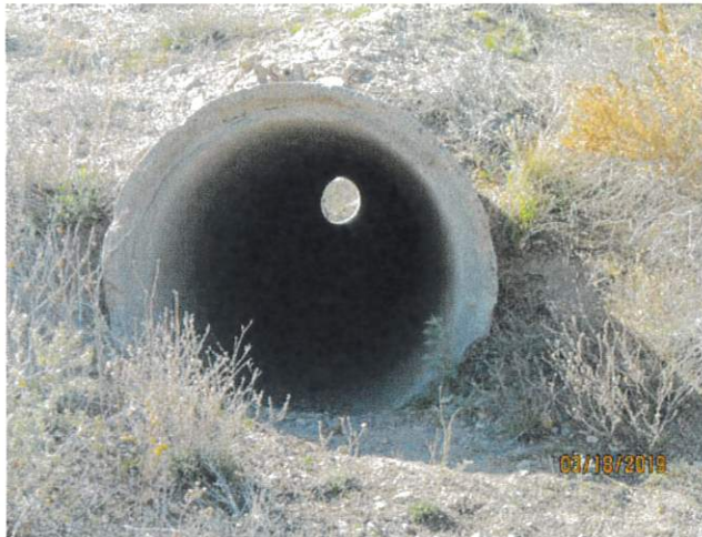
Images 14 and 15: Southerly (downstream) and northerly (upstream) views of the 36-inch diameter upper level outlet conduit.
