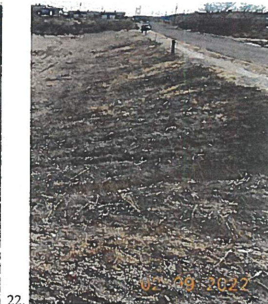
Images 21 through 23: Erosion gullies in need of repair on the upstream slope (Images 21 and 22) and more of the same on the downstream slope (Image 23).
