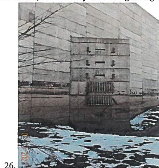
Images 26 through 28: Slightly distorted views of the low-level outlet works intake structure located at the base of the upstream face of the dam.
