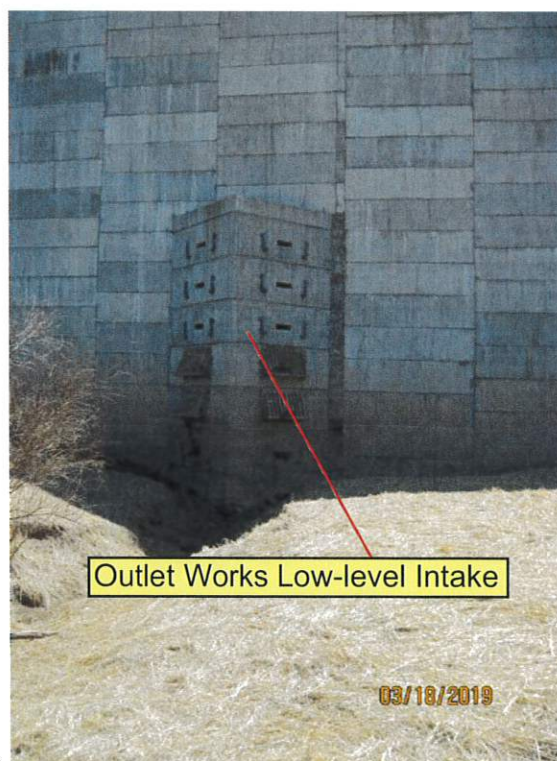
Images 33 through 35: Views emphasizing the lower-level and upper-level outlet works intakes
