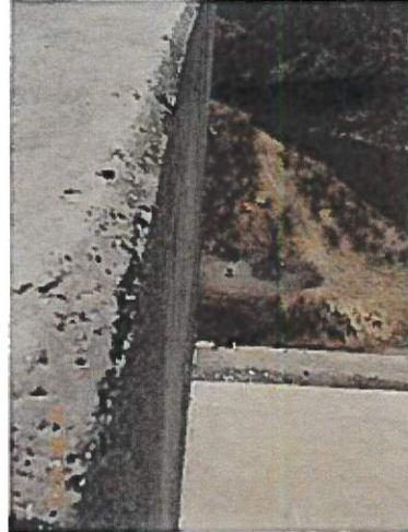
Images 20 through 22: Westerly view along the primary spillway crest (Image 20), southerly view along the left side primary spillway training wall (Image 21), and view of the lower portion of the left downstream groin of the main dam and spalled concrete at a contraction joint (Image 22).
