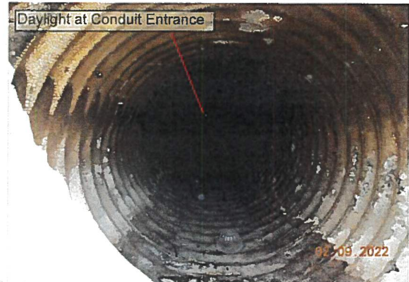
Images 14 and 15: Upstream views of the 24-inch diameter CMP outlet conduit outfall with light visible at the upstream end as indicated.
