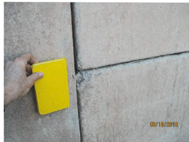
Images 47 through 50: Examples of concrete defects requiring patching at several locations on the main dam.
