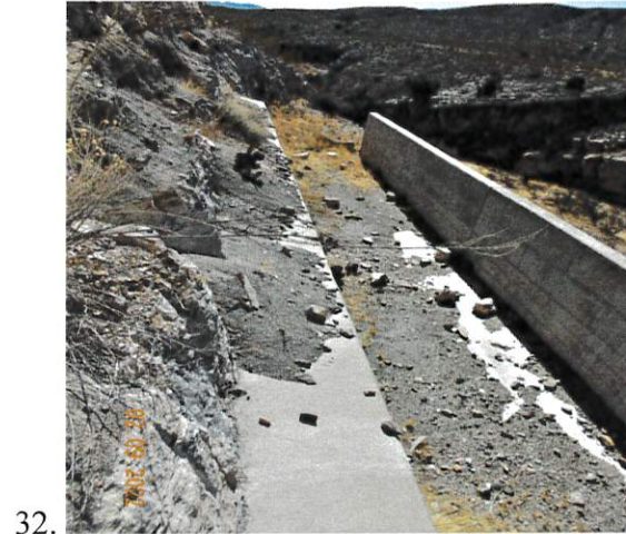
Images 31 and 32: Horizontally distorted views of the upper-level outlet works intake structure (Image 31) and concrete chute discharge channel (Image 32).
