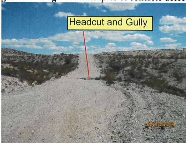
Image 51: Headcut and erosion across access road to the detention basin. Image 52: Emerging woody vegetation on the downstream face of the dam.
