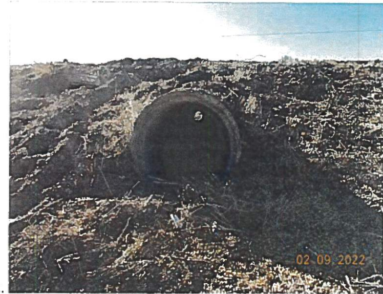
Images 11 and 12: Upstream and downstream views of the upper level outlet conduit beneath Marie Street (aka the dam crest).
