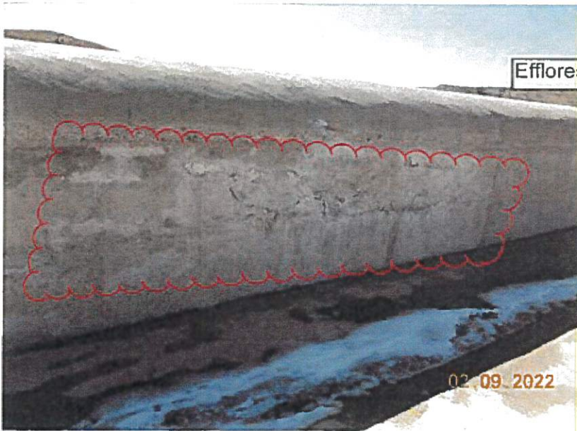
Images 37 and 38: Examples of concrete efflorescence and spalling on the upstream face of the emergency spillway ogee weir.
