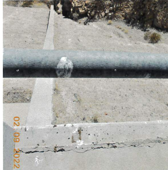
47. 48. 49. Images 47 through 49: Examples of offset joints and cracks on the upstream face, crest of the main dam and upstream face of the emergency spillway ogee section that should be monitored over time.
