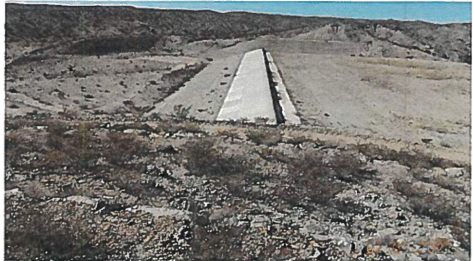
Images 33 and 34: Westerly views of the emergency spillway ogee weir located approximately 300 feet west of the right abutment of the Main Dam.
