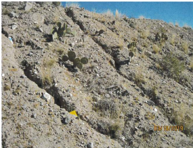
Images 9 and 10: Northerly (upstream) views of erosion on the downstream slope.
