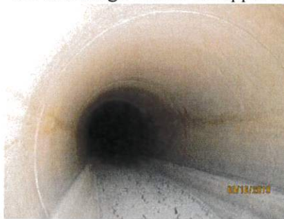
Images 42 through 44: Views of the downstream (discharge) end of the outlet works low-level conduit.
