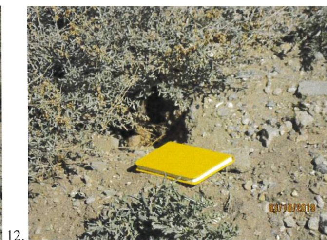
Images 11 and 12: Typical views of rodent burrows on the downstream slope.
