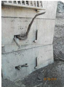
Images 36 through 38: Examples of several partially plugged ports on the outlet works lower-level intake.
