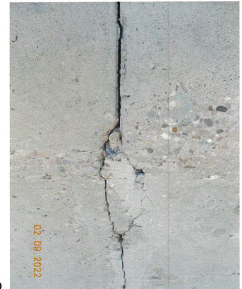
47. 48. 49. Images 47 through 49: Examples of offset joints and cracks on the upstream face, crest of the main dam and upstream face of the emergency spillway ogee section that should be monitored over time.
