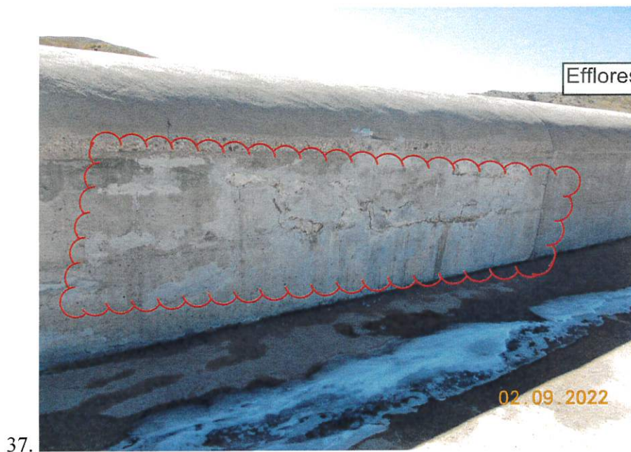
Images 37 and 38: Examples of concrete efflorescence and spalling on the upstream face of the emergency spillway ogee weir.
