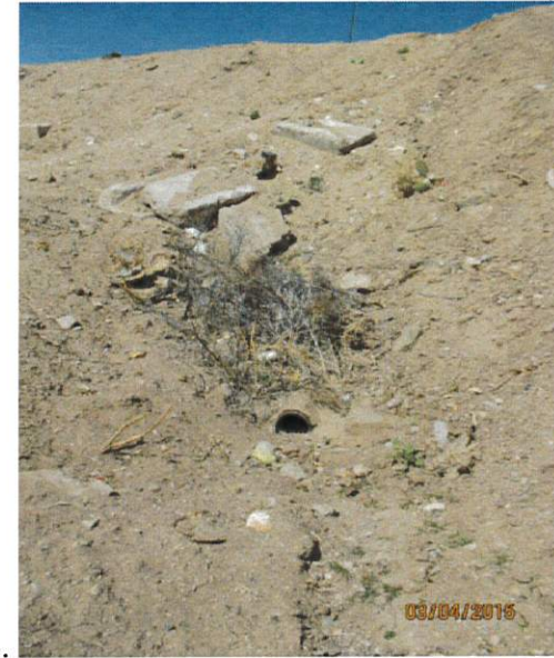
Images 13 and 14: Upstream views of the lower level outlet outfall in 2022 and 2015, respectively. The outfall is currently obscured and needs to be maintained in an exposed condition.
