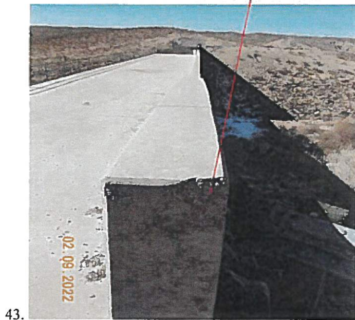
Images 41 through 44: Examples of damaged (spalled) concrete on the parapet walls of the main dam and shrinkage cracking on the crest of the main dam. Repair of the spalled concrete is required along with monitoring and documentation of the shrinkage cracks over time.
