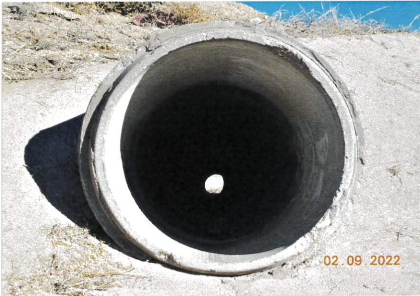
Images 11 and 12: Upstream and downstream views of the upper level outlet conduit beneath Marie Street (aka the dam crest).
