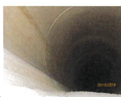
Images 42 through 44: Views of the downstream (discharge) end of the outlet works low-level conduit.
