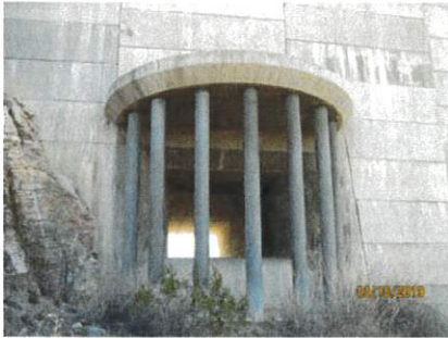
Images 39 through 41: Views of the outlet works upper-level intake, the upper-level outlet conduit, and the discharge end of the upper-level outlet conduit.
