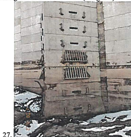
Images 26 through 28: Slightly distorted views of the low-level outlet works intake structure located at the base of the upstream face of the dam.
