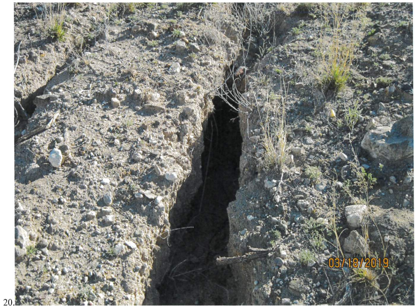
Images 18 through 20: Distant (easterly) view of erosion along the left downstream groin (Image 18), and close-up views of the same set of erosion gullies (Images 19 and 20).
