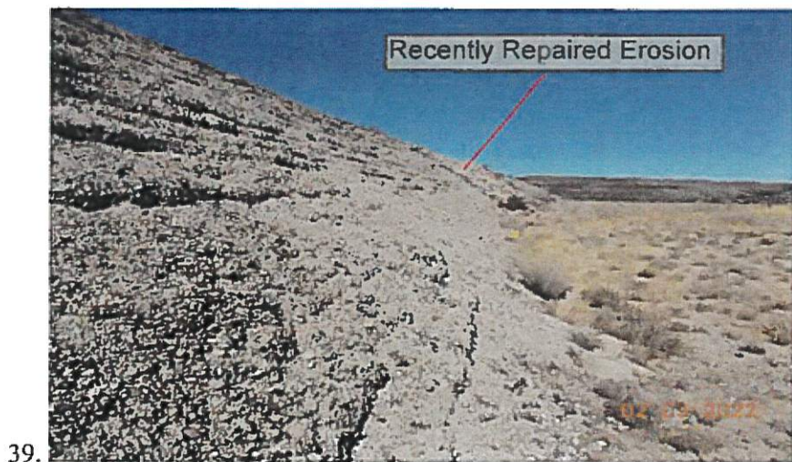
Images 39 and 40: Views of soil cement armoring on right side slope of emergency spillway approach channel (Image 39) and armoring on the downstream slope of the emergency spillway ogee section.
