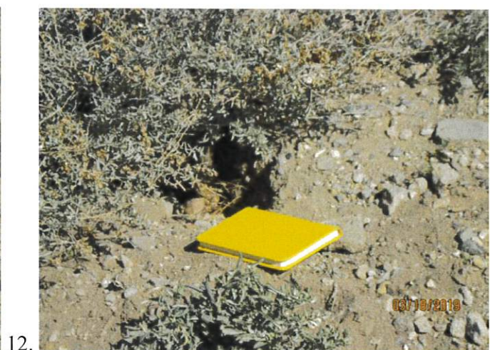
Images 11 and 12: Typical views of rodent burrows on the downstream slope.
