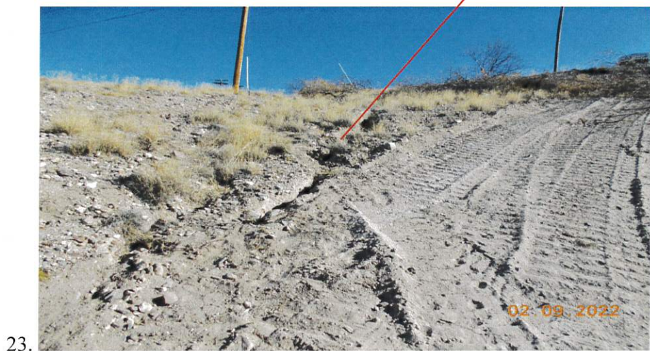
Images 21 through 24: Views of past off-road vehicle (ORV) traffic on the upstream slope (Images 21 and 22) and erosion gullies on the downstream slope (Images 23 and 24).
