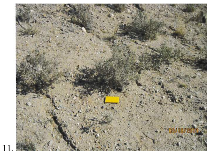
Images 11 and 12: Typical views of rodent burrows on the downstream slope.
