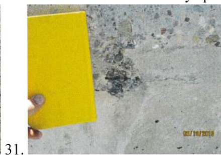
Images 30 through 32: Typical views of details pertaining to the auxiliary spillway; RCC degradation on the downstream stepped section of the spillway (Image 30), deterioration of one of several patched portions of upstream face of the ogee section (Image 31), one of several daylighted drain outfalls on the downstream face auxiliary spillway (Image 32).
