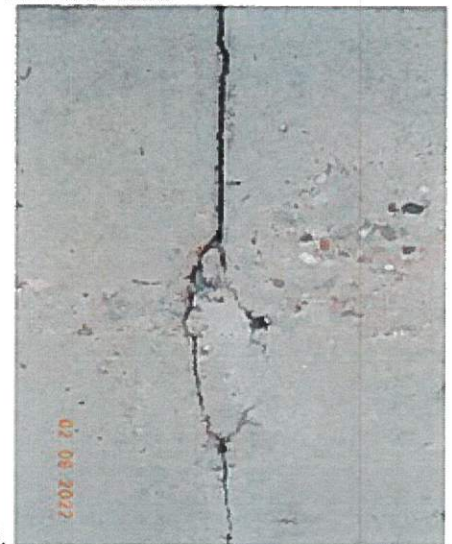
Images 47 through 49: Examples of offset joints and cracks on the upstream face, crest of the main dam and upstream face of the emergency spillway ogee section that should be monitored over time.
