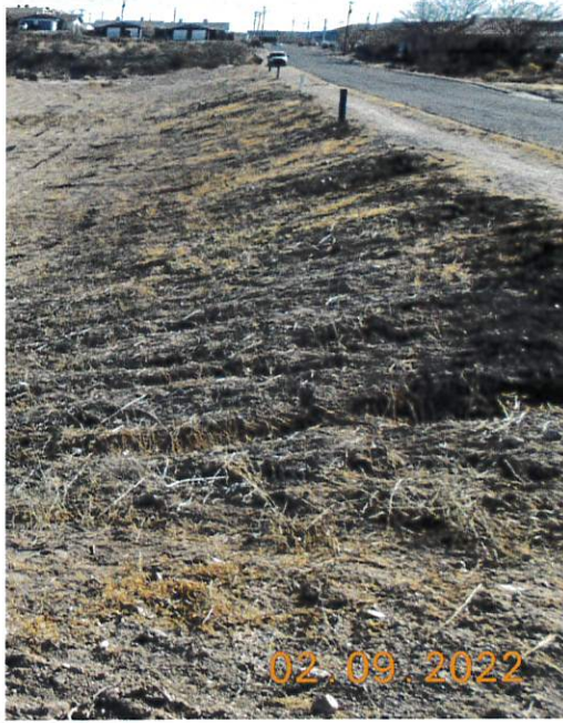
Images 21 through 23: Erosion gullies in need of repair on the upstream slope (Images 21 and 22) and more of the same on the downstream slope (Image 23).
