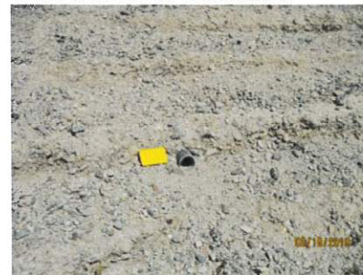
Images 30 through 32: Typical views of details pertaining to the auxiliary spillway; RCC degradation on the downstream stepped section of the spillway (Image 30), deterioration of one of several patched portions of upstream face of the ogee section (Image 31), one of several daylighted drain outfalls on the downstream face auxiliary spillway (Image 32).
