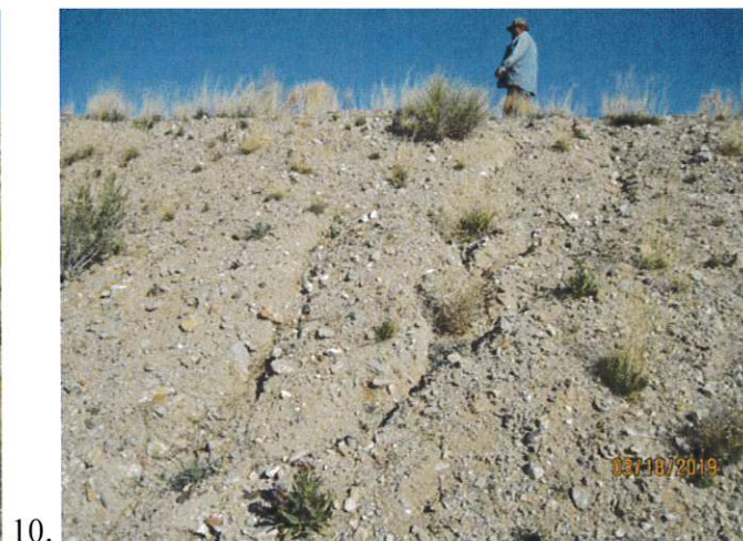
Images 9 and 10: Northerly (upstream) views of erosion on the downstream slope.
