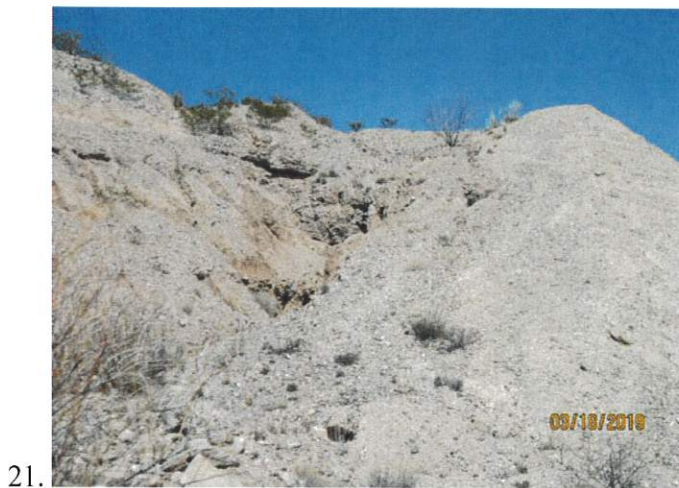
Images 20 through 22: Aerial view from GoogleEarth (Image 20) of large erosion gully located along the soil cement armored right abutment of the auxiliary spillway; additional views of the same erosion gully seen from ground level (Images 21 and 22).
