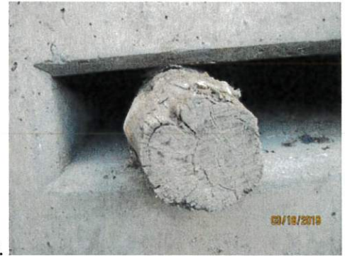
Images 36 through 38: Examples of several partially plugged ports on the outlet works lower-level intake.
