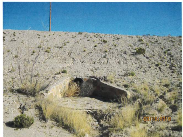
Images 13 through 15: Southerly (downstream) view of the outlet conduit intake (Image 13), close-up view of the outlet intake (Image 14), and northerly (upstream) view of the outlet conduit outfall (Image 15).
