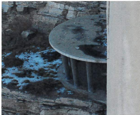
Images 31 and 32: Horizontally distorted views of the upper-level outlet works intake structure (Image 31) and concrete chute discharge channel (Image 32).
