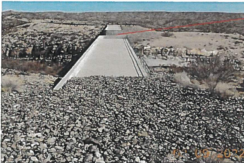
Images 5 and 6: Easterly view of the west end of the dam crest (Image 5) as seen from the vicinity of the right abutment and upstream (northerly) view (Image 6) of the downstream face of the main dam at the primary spillway overpour section.
