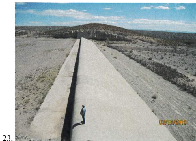
Images 23 and 24: Easterly and westerly views along the ogee crest of the auxiliary spillway, respectively.
