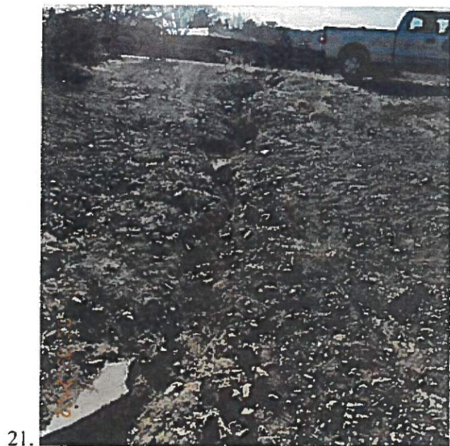
Images 21 through 23: Erosion gullies in need of repair on the upstream slope (Images 21 and 22) and more of the same on the downstream slope (Image 23).
