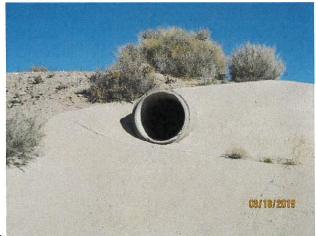
Images 14 and 15: Southerly (downstream) and northerly (upstream) views of the 36-inch diameter upper level outlet conduit.
