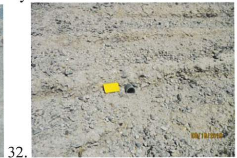
Images 30 through 32: Typical views of details pertaining to the auxiliary spillway; RCC degradation on the downstream stepped section of the spillway (Image 30), deterioration of one of several patched portions of upstream face of the ogee section (Image 31), one of several daylighted drain outfalls on the downstream face auxiliary spillway (Image 32).
