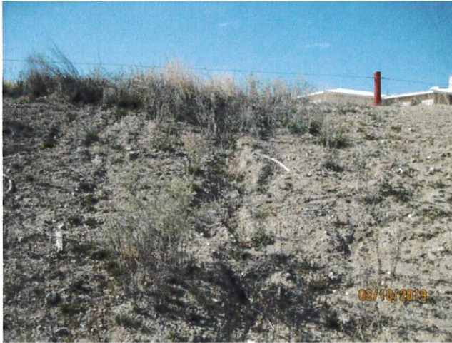
Images 13 and 14: Southerly views of erosion typical to the upstream slope and the area downstream of the dam, respectively.
