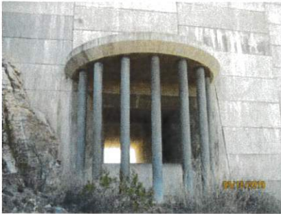
Images 39 through 41: Views of the outlet works upper-level intake, the upper-level outlet conduit, and the discharge end of the upper-level outlet conduit.
