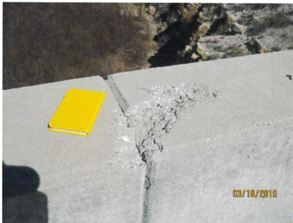
Images 47 through 50: Examples of concrete defects requiring patching at several locations on the main dam.
