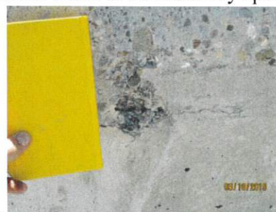
Images 30 through 32: Typical views of details pertaining to the auxiliary spillway; RCC degradation on the downstream stepped section of the spillway (Image 30), deterioration of one of several patched portions of upstream face of the ogee section (Image 31), one of several daylighted drain outfalls on the downstream face auxiliary spillway (Image 32).
