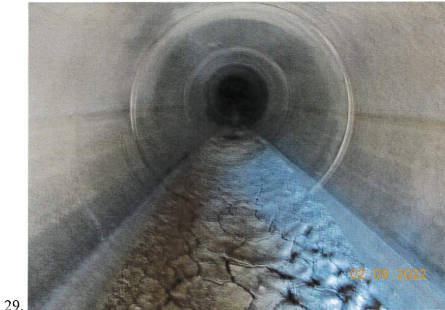
Images 29 and 30: Upstream interior views of the low-level outlet conduit as seen from the discharge end of the conduit. The upstream end of the conduit is located at the upstream face of the dam and within the outlet works structure shown in Images 26 through 28.
