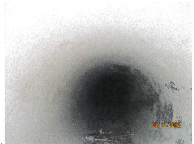
Images 16 and 17: Views of the 8-inch diameter lower level outlet conduit outfall and interior view of the same outlet conduit, respectively.
