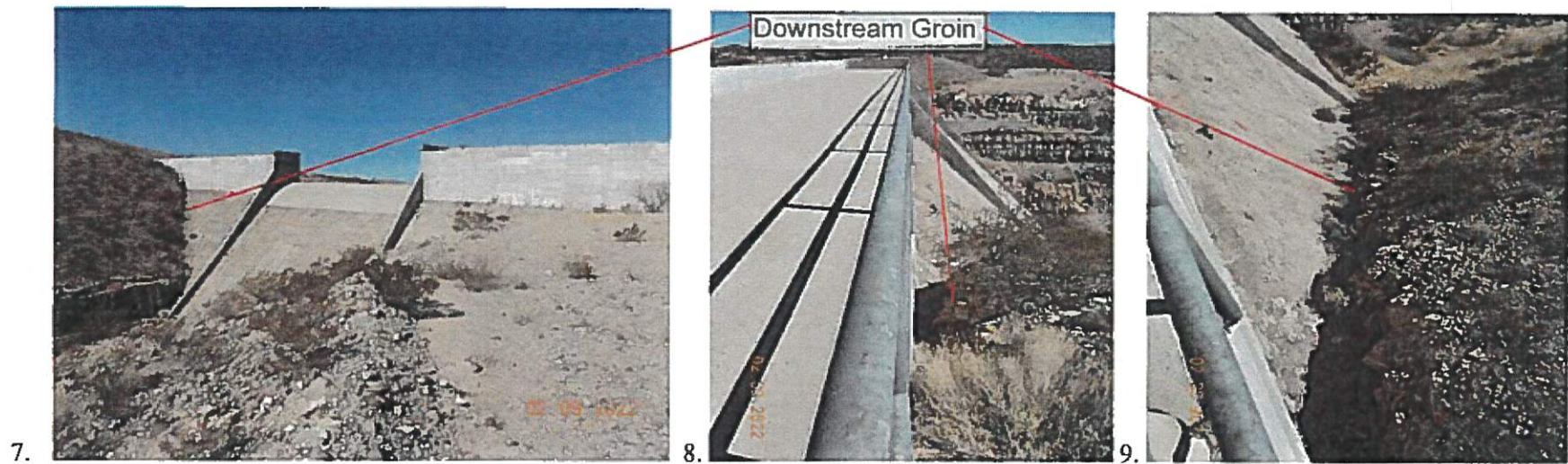
Images 7 through 9: Westerly view of the downstream slope of the main dam (Image 7) and easterly views along the downstream shoulder of the dam crest and the lower section of the right downstream groin (Images 8 and 9).
