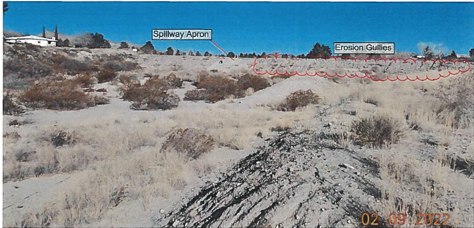
Image 8: Northerly view of the downstream slope with areas of erosion and spillway apron as indicated.
