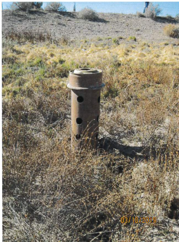
Images 20 and 21: Additional view of the low level outlet works riser (Image 20) and interior view of the riser (Image 21) with plugged ports as an approximate indication of the sediment level.
