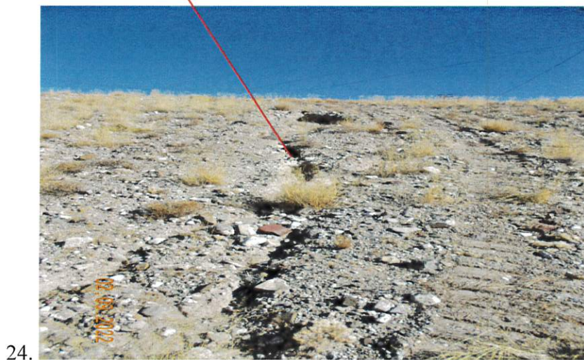
Images 21 through 24: Views of past off-road vehicle (ORV) traffic on the upstream slope (Images 21 and 22) and erosion gullies on the downstream slope (Images 23 and 24).
