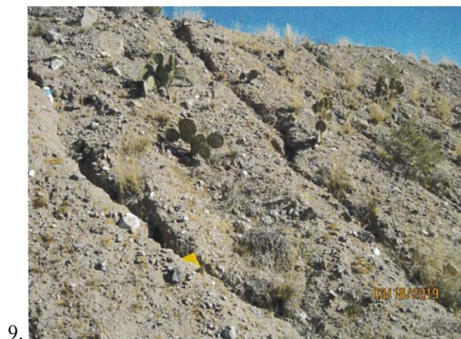
Images 9 and 10: Northerly (upstream) views of erosion on the downstream slope.
