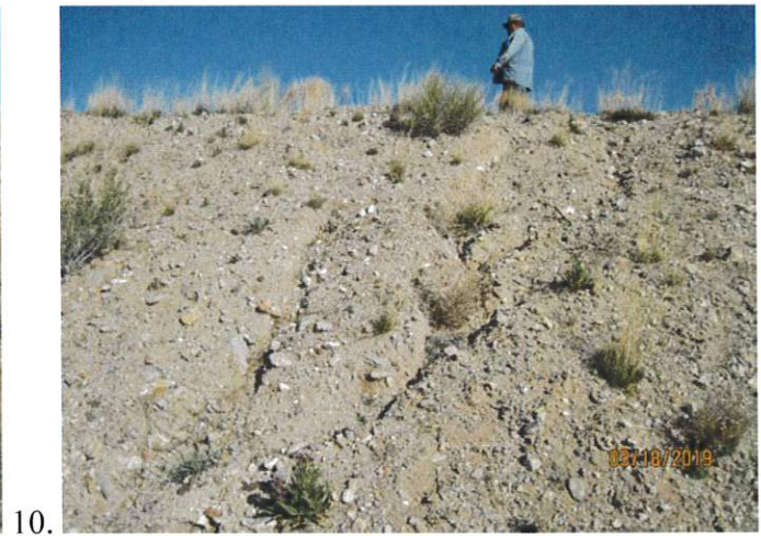
Images 9 and 10: Northerly (upstream) views of erosion on the downstream slope.
