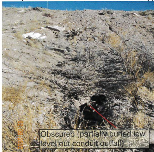
Images 13 and 14: Upstream views of the lower level outlet outfall in 2022 and 2015, respectively. The outfall is currently obscured and needs to be maintained in an exposed condition.
