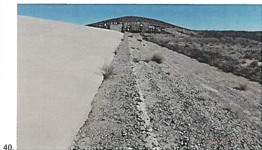
Images 39 and 40: Views of soil cement armoring on right side slope of emergency spillway approach channel (Image 39) and armoring on the downstream slope of the emergency spillway ogee section.
