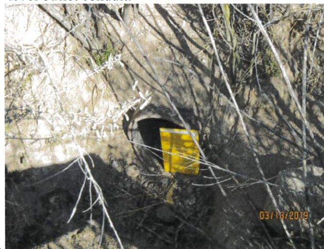
Images 16 and 17: Views of the 8-inch diameter lower level outlet conduit outfall and interior view of the same outlet conduit, respectively.
