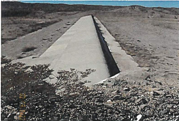
Images 33 and 34: Westerly views of the emergency spillway ogee weir located approximately 300 feet west of the right abutment of the Main Dam.
