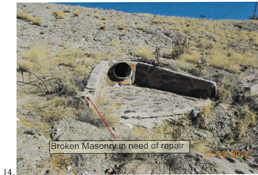
Images 14 and 15: Upstream views of the 24-inch diameter CMP outlet conduit outfall with light visible at the upstream end as indicated.
