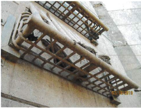
Images 36 through 38: Examples of several partially plugged ports on the outlet works lower-level intake.
