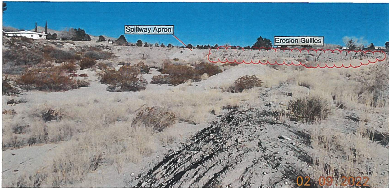
Image 8: Northerly view of the downstream slope with areas of erosion and spillway apron as indicated.
