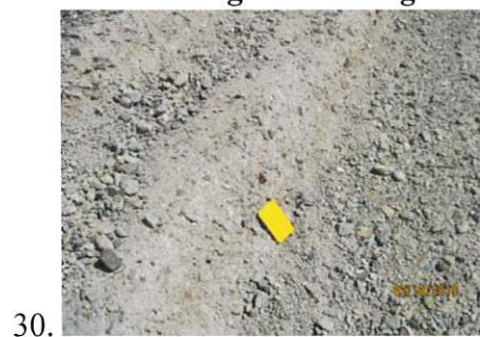
Images 30 through 32: Typical views of details pertaining to the auxiliary spillway; RCC degradation on the downstream stepped section of the spillway (Image 30), deterioration of one of several patched portions of upstream face of the ogee section (Image 31), one of several daylighted drain outfalls on the downstream face auxiliary spillway (Image 32).
