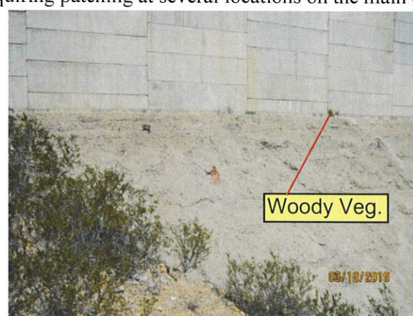
Image 51: Headcut and erosion across access road to the detention basin. Image 52: Emerging woody vegetation on the downstream face of the dam.
