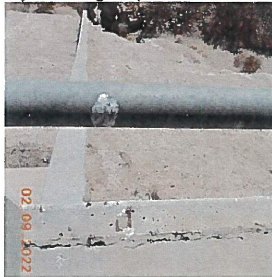
Images 47 through 49: Examples of offset joints and cracks on the upstream face, crest of the main dam and upstream face of the emergency spillway ogee section that should be monitored over time.
