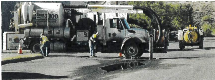
Street Crew repairs a leak
