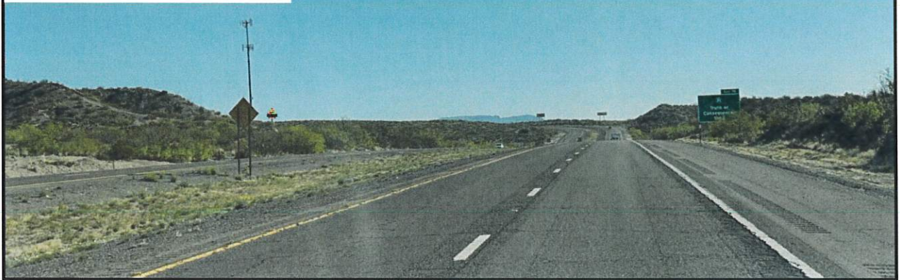
NORTHBOUND 1.0 MILE FROM EXIT
