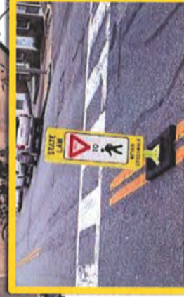
Figure 96: R1-6 Pedestrian gateway treatment.
